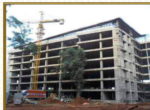
Construction of Multi-storeyed IT Block at Infopark Thrissur in Progress.
